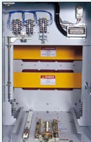
Circuit Breaker Removed
